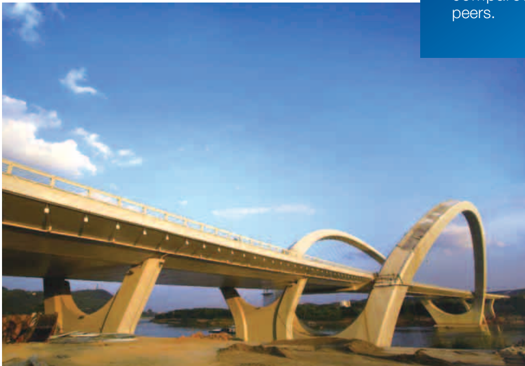
Nanning Bridge, the first long span suspension bridge in the world constructed under the support of the Group.
