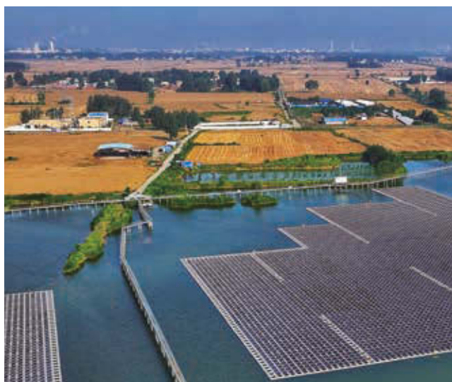
▲ The Bank's Anhui Branch supported the green finance project of Suzhou Floating Photovoltaic Power Station
